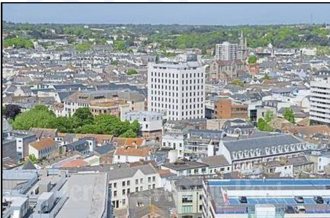
Figure 2: Urban context (aerial view from south-east)
